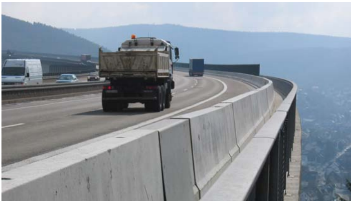
Figure 1: Premium bridge restraint system Delta Bloc 100 AS-R, containment level H4b, Siegtal bridge - Germany
